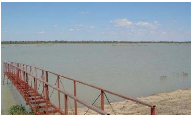
Ring tank – irrigation water storage structure
